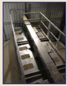
standard 29tph drier, so an integral hopper was installed to keep the height of the drier down. Also as the drier is in a building the fans had to be side mounted to ensure the air was not directed over a roof or towards other building walls. The fans were fitted with dust shutters to minimise the amount of dust and chaff that leaves the drier when it discharges.
